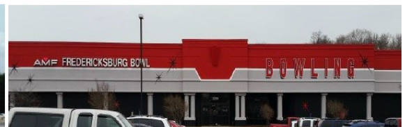
AMF Fredericksburg Lanes
