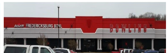
AMF Fredericksburg Lanes
